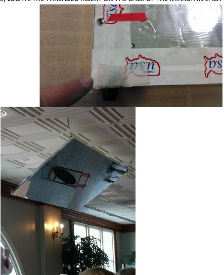
4) THREAD EYEBOLT INTO EACH CORNER AND TIGHTEN LOCK NUT WITH WRENCH
